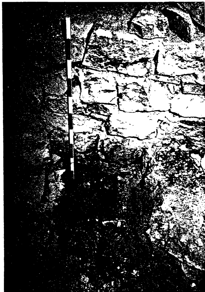
Figure 14. Detail of west side of center wall. (Photo by author; 24H-973M)
